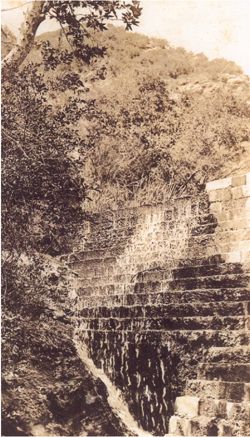
This is a dam in Harding Canyon that S.J. Finley designed and built in 1900. This dam brought water down pipes to the pool at the Modjeska House. The water was used to irrigate the plants on the property.
